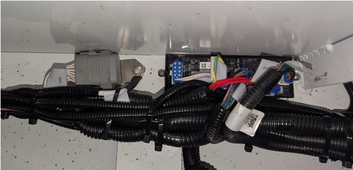
Figure 32: Tunnel Box Panel
